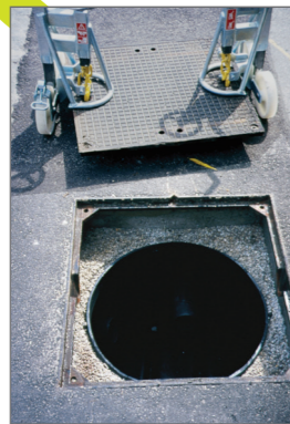
Watertight chamber cover system with separate sealing and load-bearing function
