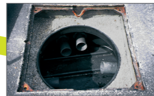
Watertight chamber cover system with separate sealing and load-bearing function
