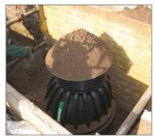
After then pour the backfilling material on the lid, wherein the backfilling material is distributed around the manhole and the manhole is protected from contamination. Now remove upper unit and assemble next component in accordance with 3.3.
