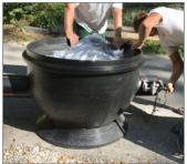
All PE spigot ends have to be pre-cleaned, the pipe end checked for perpendicularity, cutting edges to be deburred and sawdust removed.
