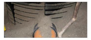
The backfilling material is to be inserted carefully and in layers of 20–40 cm layer thickness and compacted with a medium vibrating stamper (approx. 50kg).
