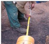
The support area of the manhole base must be established in accordance with the planning (differential between base to channel level = 20 cm).
