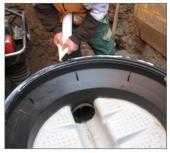
Align all manhole elements in acordance with vertical marks to ensure the vertical alignment of the ladder.
