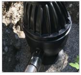
The oxide layer has to be scraped away properly. We recommend the use of a eotational scraper tool. Clean all pipe ends with PE-cleaner, mark insertion depths, push in sockets and weld without causing tension. Installation instructions of the socket manufacturer must be observed!
