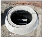
If needed, the upper unit seal is to be mounted on the upper unit neck before assembling the concrete ring and seal with sufficient lubricant. The concrete support ring must be set up centrally without affecting the bedding.
