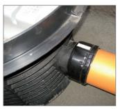
The inserted seals should be checked for correct fitting and inspected for damage, cleaning may be necessary.
