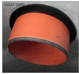
Drill with an electric hand drill at the desired position with a ROMOLD cup saw the total possible drilling depth. Drilling in the area of the base – riser pipe connection is not allowed. Deburr hole and insert the seal from the outside without using lubricant, the collar of the seal is up to the ribs at the outside of the riser pipe. Lubricate the spigot end of the pipe as well as the inside of the seal and insert the pipe creating an inner overlap afterwards.
