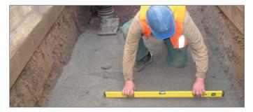
The support area of the manhole base must be load-bearing and completely levelled. The support area of the manhole base must be established in accordance with the planning specifications (difference between base and channel level = 5 cm).
