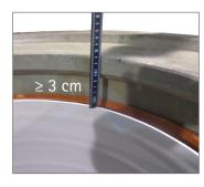
If needed, the seal is to be mounted on the chamber neck before assembling the concrete ring and seal with sufficient lubricant. The concrete support ring must be set up centrally without affecting the bedding. The concrete support ring is covered with a steel plate until the
