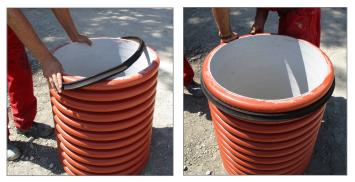
installation of the cover. The total height of the concrete support ring and commercial cover class D 400 is about 30 cm (without using a height adjustment ring AR-V  $625 \times 60$  mm) from the upper edge of the PP riser pipe.
