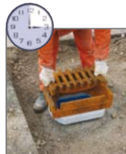
15. Min.: assembly of grating
