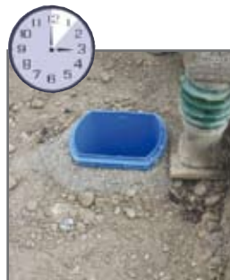
7. Min.: backfilling and compacting
