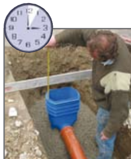
5. Min.: height adjustment
