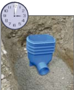
3. Min.: bedding in lean concrete mix
